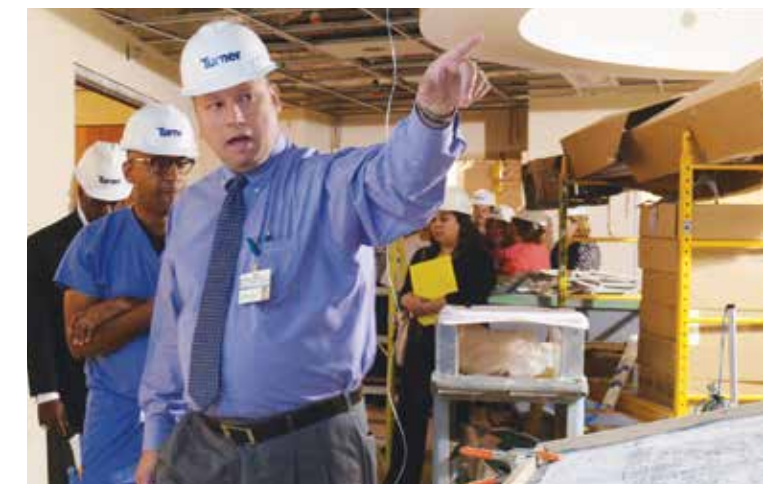
Brandon Sternbach, Administrative Director of Plant Operations and Construction at Aria Health, touring EMS and Aria staff through the newly constructed Torresdale Campus Emergency Department.
